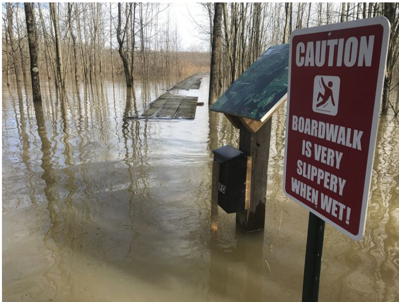
John Lawrence | Late February rains led to flooding in Monroe County, including along the boardwalk path into Beanblossom Bottoms Nature Preserve in Monroe County. The boardwalk in the flooded area will soon be replaced. Work will begin on March 26 and temporarily will close the popular nature preserve to visitors.
